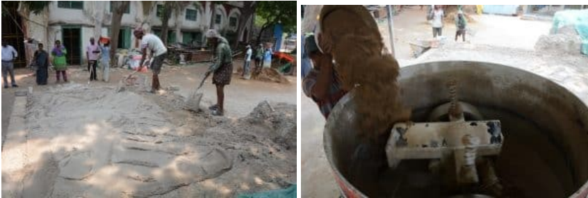
Fig – 03 – Preparation of plaster at Chepauk palace
