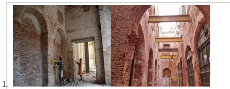
Fig.2. – Complete removal of plaster from walls
