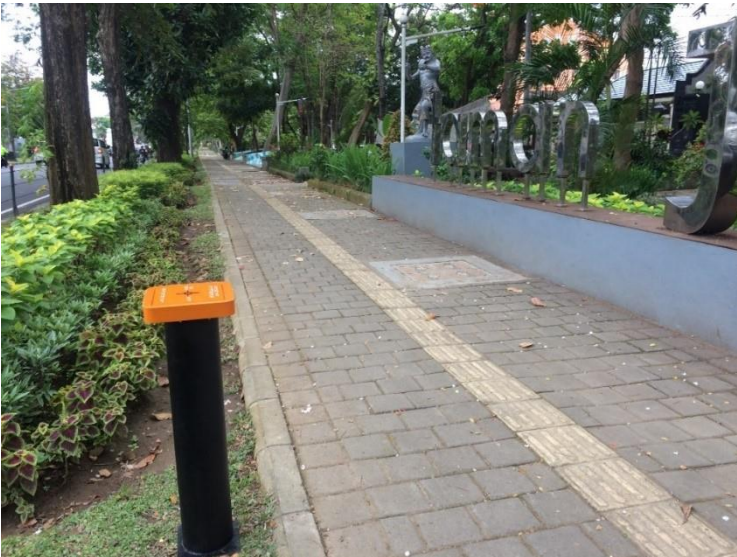
Figure 6. Guiding Blind with braille location guidance and integrated NFC RFID tag placed on the pedestrian path
