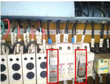
Figure 3: Adding Fuse and Holder
