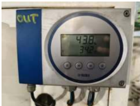
Figure 4. Hydrogen Humidity After Dryer
