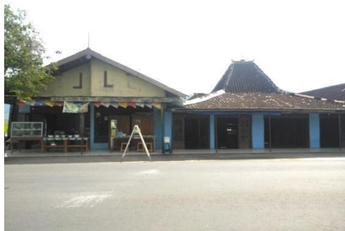
Figure 1. Existing the Joglo House.
