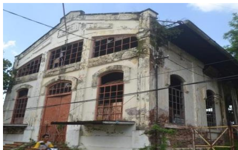
Fig. 5. The 103-year-old Central Building
