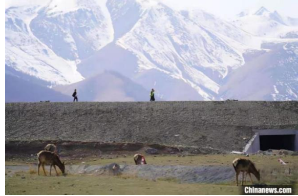
Figure 2 G575 culverts connect mountain forests and grasslands in Xinjiang, China
